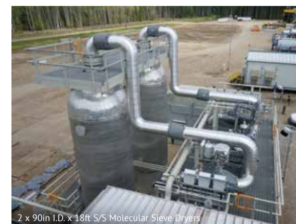
600 gpm Amine Gas Sweetening Train, 150 MMSCFD
