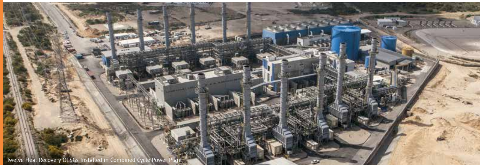
Twelve Heat Recovery OTSGs Installed in Combined Cycle Power Plant
