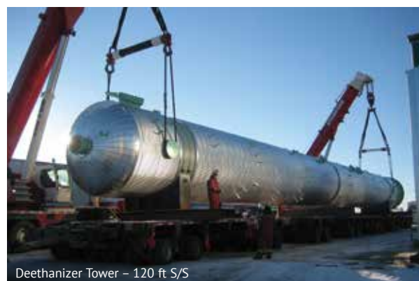
Deethanizer Tower – 120 ft S/S
